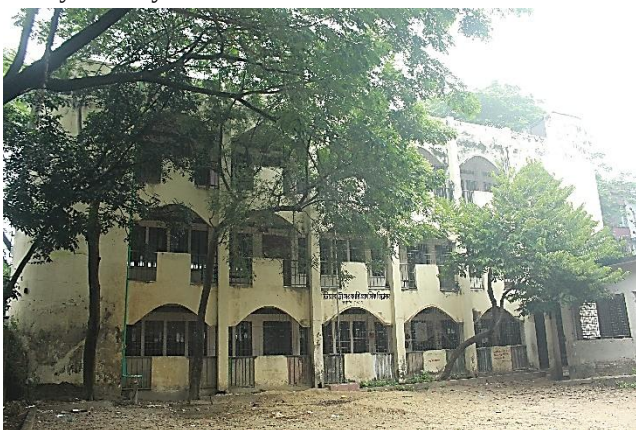
Figure 3: View of the school from the playground
