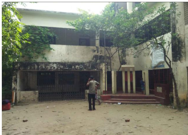
Figure 2: View of the school from the playground
