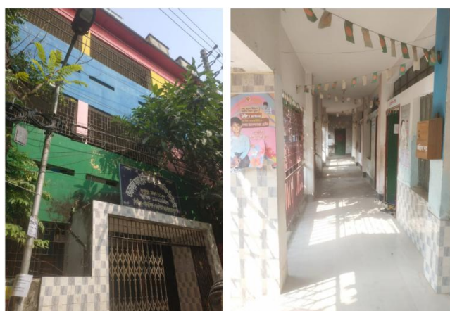
Figure 9: View from the entrance and corridor
