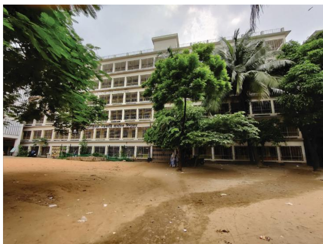
Figure 8: View from the playground of the building
