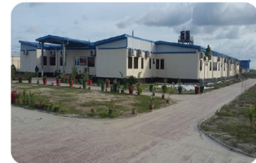
Prefabricated Building construction at Rampal Thermal Power Plant
