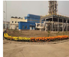
Gazipur 105 MW HFO Fired Power Plant
