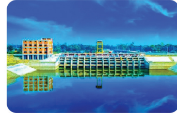
Talimnagar Pump House, Pabna
