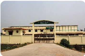
Cold Storage construction at Kurigram
