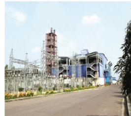
Raozan 25 MW Dual-Fuel Power Plant
