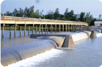
Rubber Dam construction Project at Cox's Bazar
