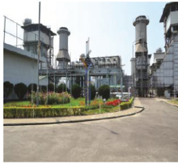
Mymensingh 210 MW Power Station
