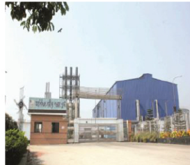
Gazipur 52 MW Dual-Fuel Power Plant
