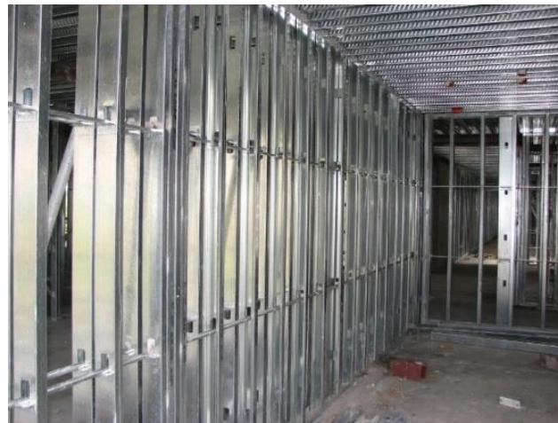
Figure 1.4: Cold-formed steel in walling (Allen, 2022)
