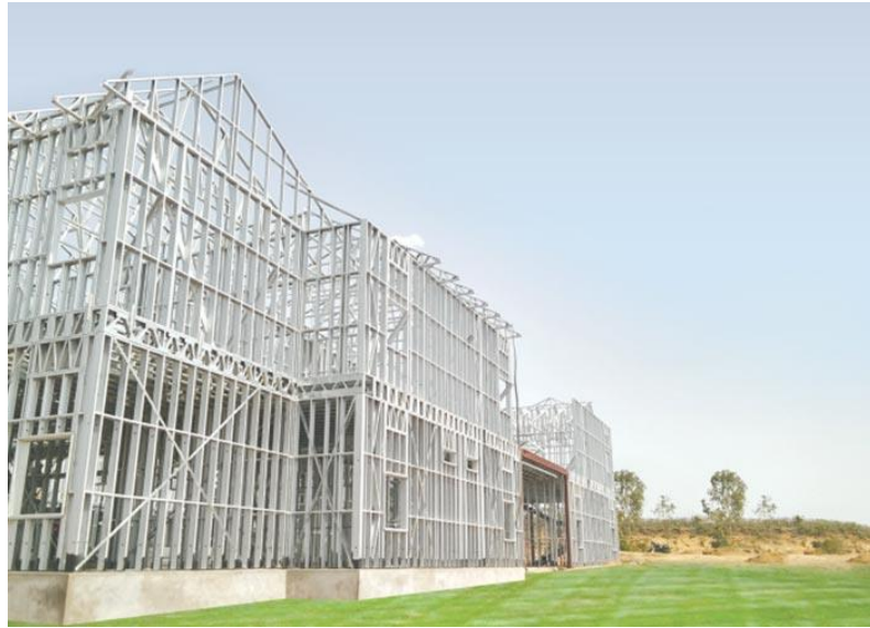
Figure 1.3: Cold form steel in the frames of houses (Barnard, 2011)
