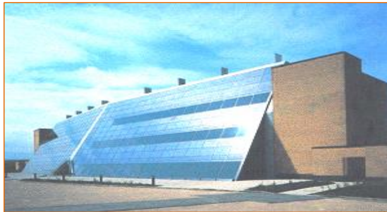
Figure 2.15: PV facade of the Solar Office at Doxford International, Sunderland, U.K. [7]
