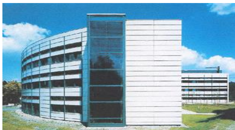
Figure 2.14: The PV Façade at the Office Building of the Fraunhofer ISE ,Freiburg[7]
