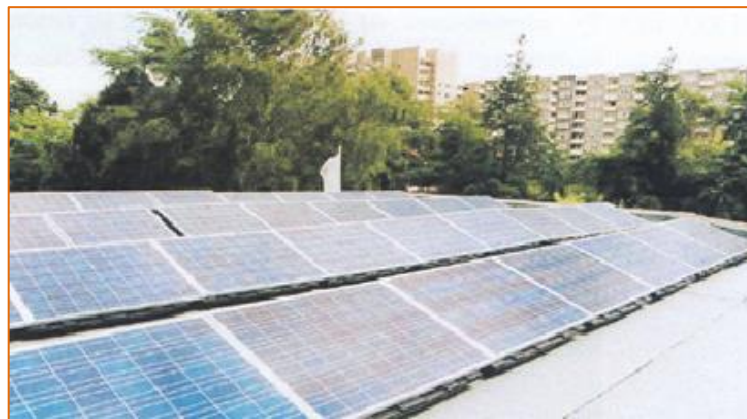
Figure 2.12: Example of an Installation on a Flat Roof
