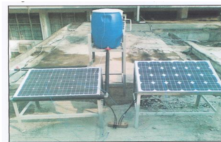
Figure 7.6: The Experimental set-up for the water cooling system
