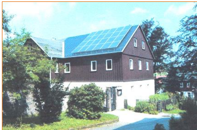
Figure 2.11: Example of an installation on a slope roof [6]
