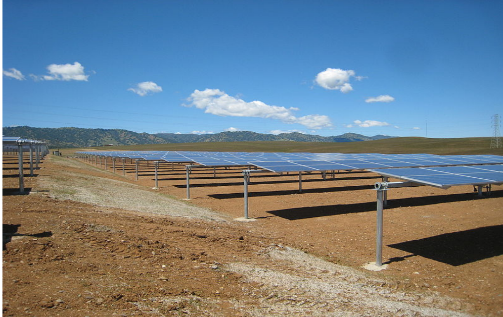
Figure 6.1 : Horizontal single axis tracker in California [37]
