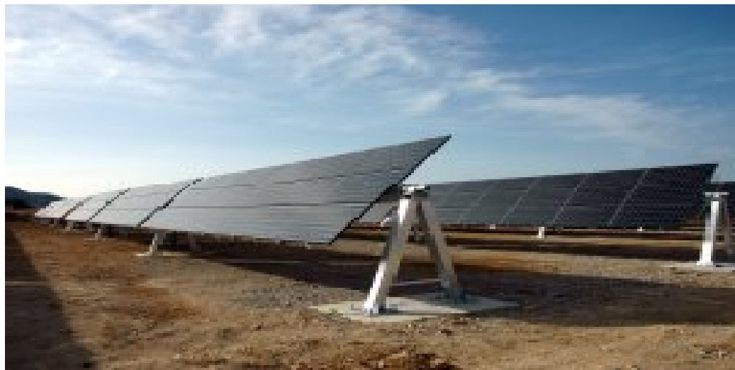
Figure 6.2 : Linear horizontal axis tracker in South Korea.[38]
