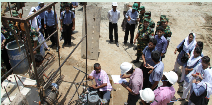
Students of Civil Engineering Batch-12 visited Mirpur-Airport Road Flyover Project and Hatirjheel Project of 16 Engineer Construction Battalion on 7 Jul 2012.
