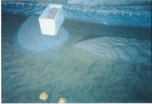
Fig 22. Apron material on the downstream side of protected structure
