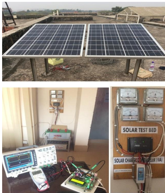
Fig. 5.17 Experimental setup of the designed solar charge controller
