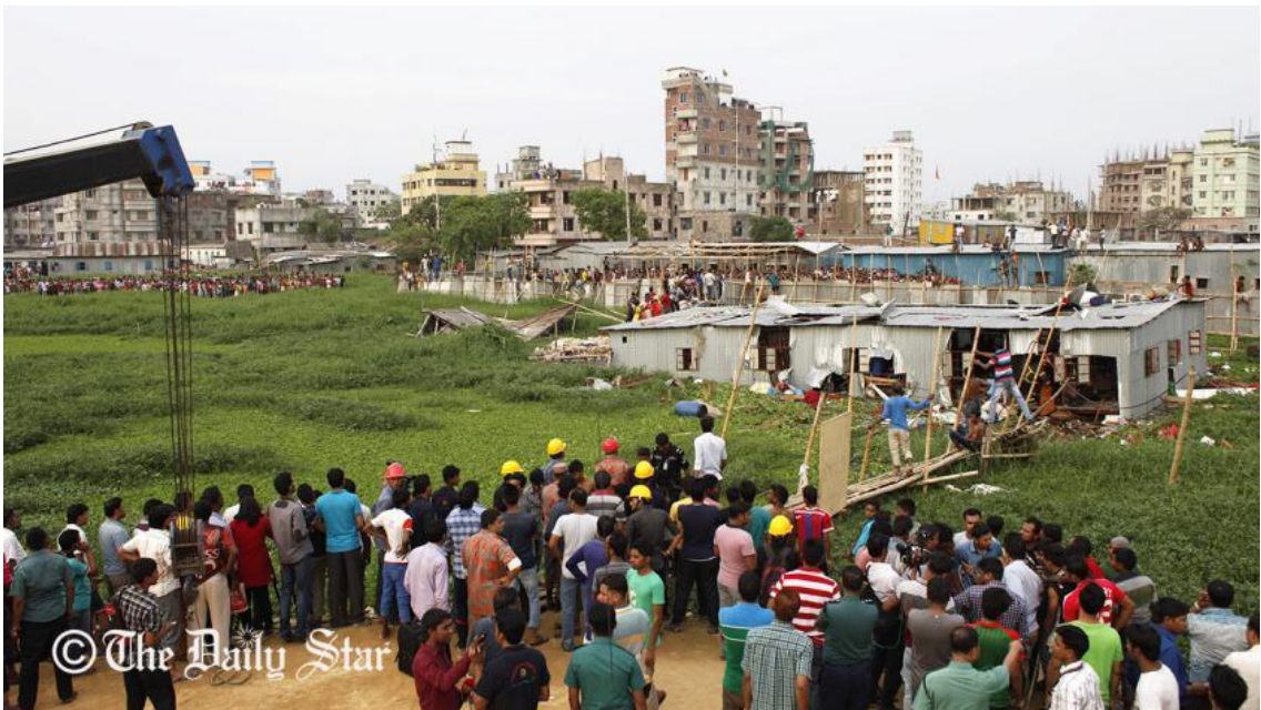
(b) Rampura building collapse killing 12 person.
