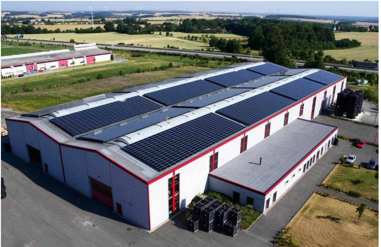
Fig. 1.5: PV Panels in Industries
