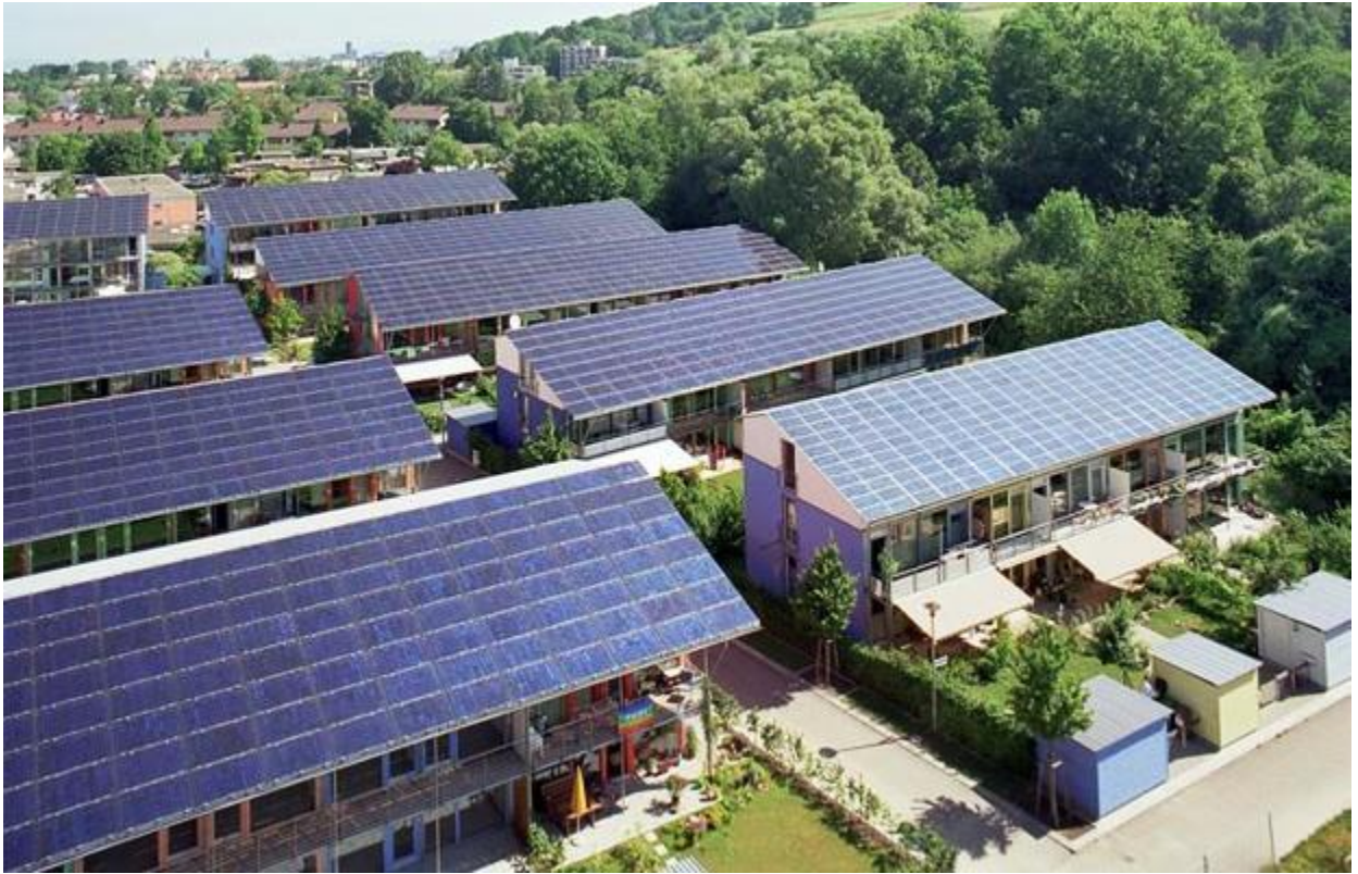
Fig.1.6: PV Panels in Residential Area
