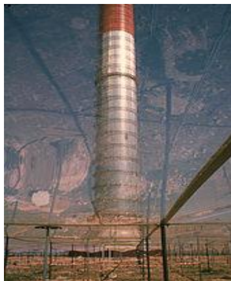
Figure 23: Manzanarez solar Chimney,Spain
