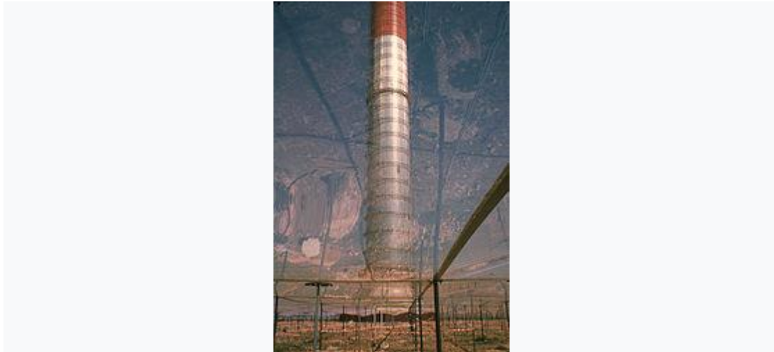
Figure 7:Manzanares solar chimney viewed through the polyster collector roof
