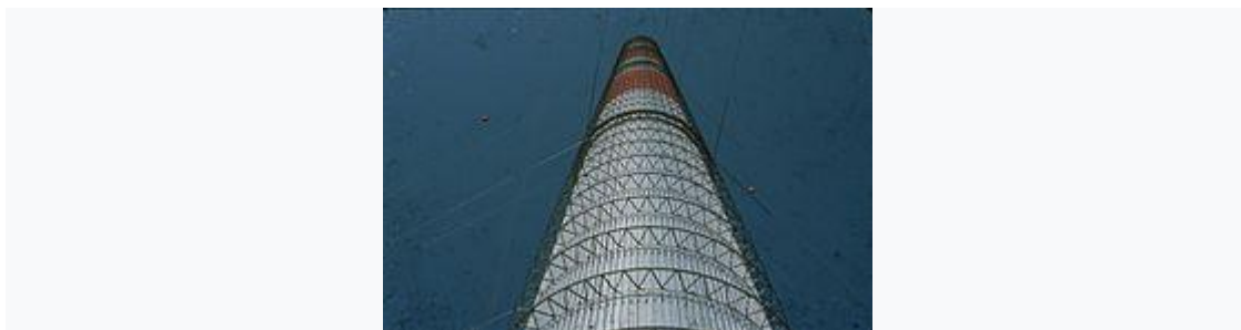
Figure 10: Manzanares Solar Chimney-view of the tower through the collector glass roof
