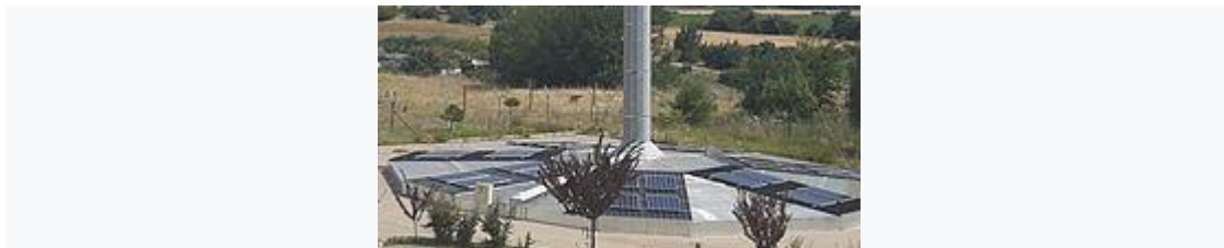
Figure 12: Solar tower incorporate photovoltaic modules on transpired collector
