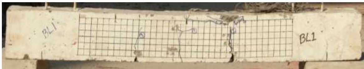
(a) Observed beam specimen
