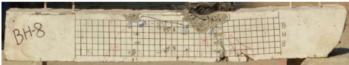
(a) Observed beam specimen
