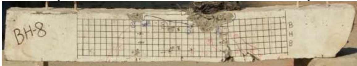
Fig 4. 24: Failure Mode for beam SSH- 2 due to concrete crushing
