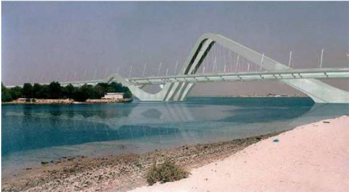
Fig 1. 2 : Sheik Zayed bridge in Abu Dhabi. Adopted from Rabi, Cashell et al. 2019 [15]
