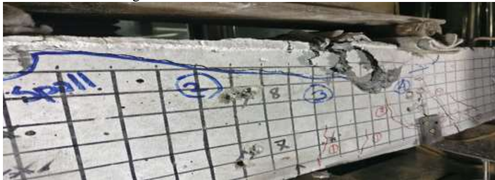
Fig 4. 18 : Crack Pattern for beam SSH-2
