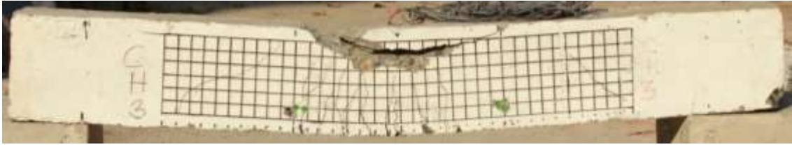
(a) Observed beam specimen
