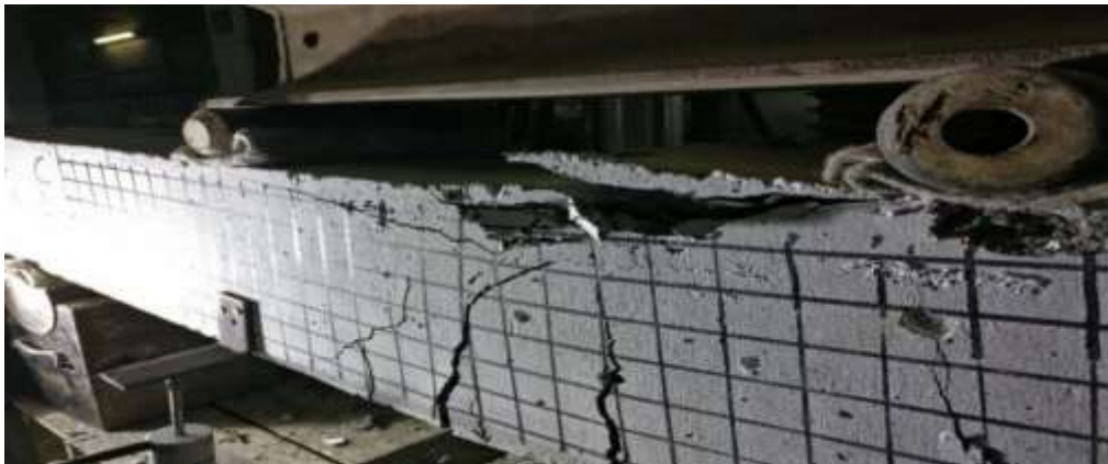
Fig 4. 3 : Crack Pattern for beam MSL-1
