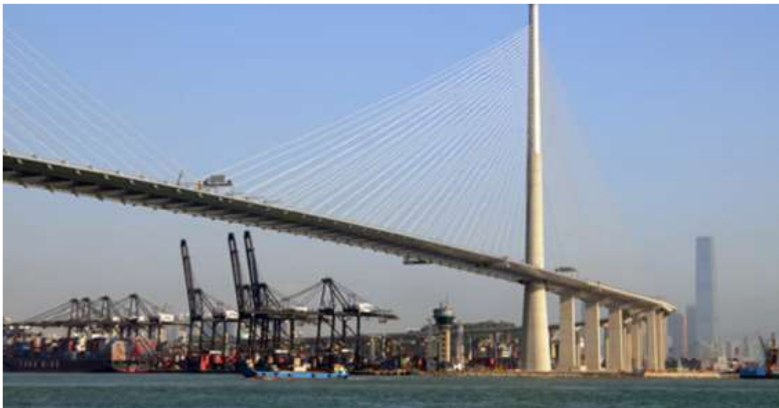
Fig 1. 1: Stonecutters bridge in Hong Kong. Adopted from Rabi, Cashell et al. 2019[15]
