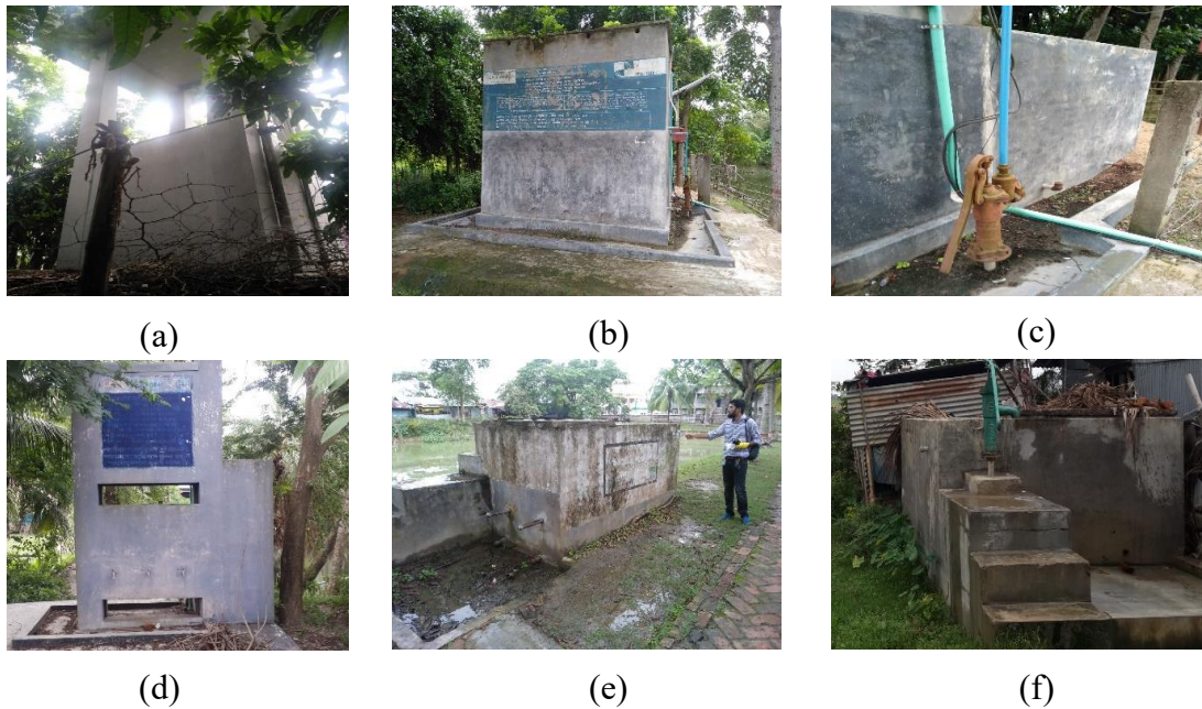
Fig. 4.8. Pond Sand Filters (PSFs) in different unions of Mongla Upazila; (a) Chandpi, (b) Chila, (c) Sundarban, (d) Suniltala, (e) Mithakhali and (f) Burirdanga
