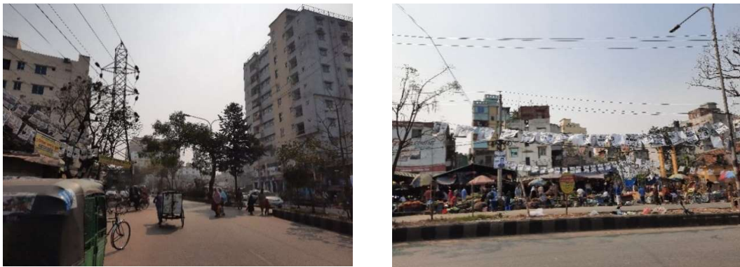
Figure 3.9: Existing Condition of Ranikhola Bazar, Shah Ali
