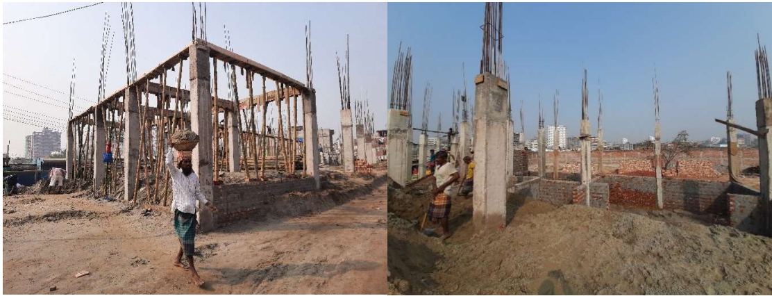
Figure 3.5: Existing condition of Bosila Area, Mohammadpur
