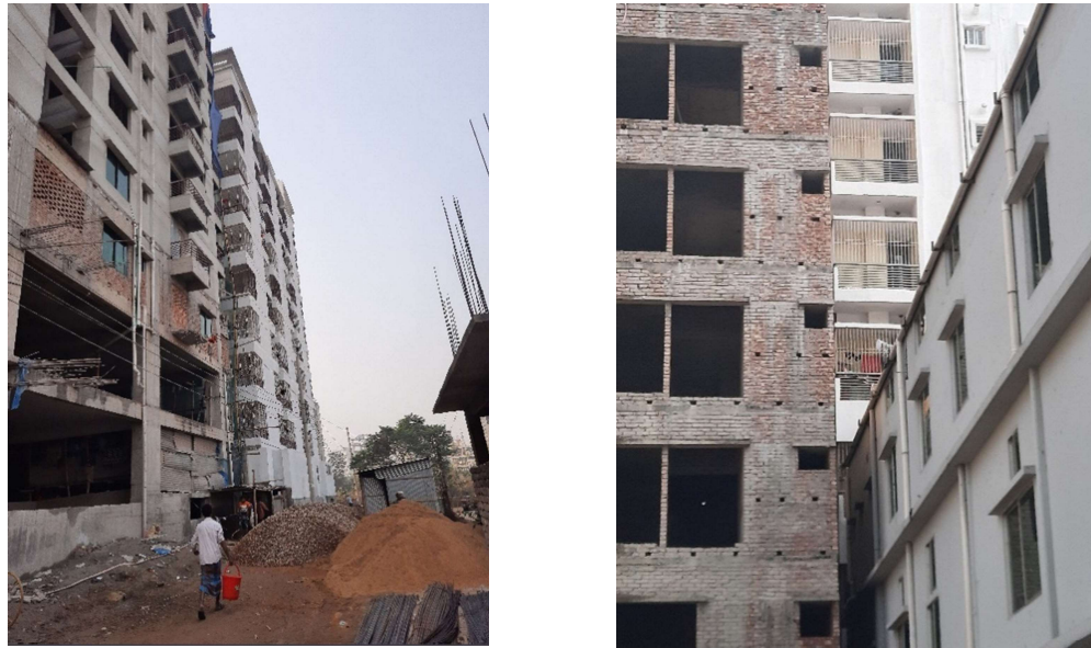
Figure 3.6: Existing Condition of Kedarabad Housing, Mohammadpur
