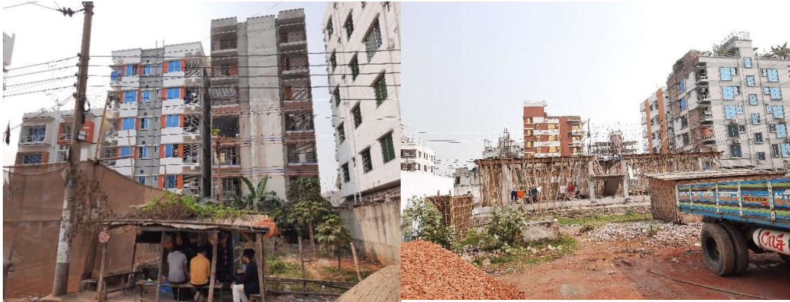
Figure 3.10: Existing Condition of Eastern Housing, Mirpur
