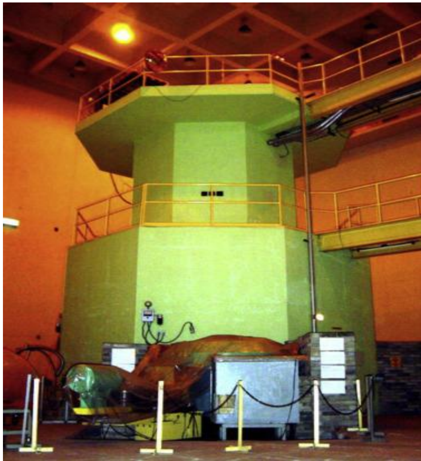
Figure 3. 5: TRIGA MARK-II research reactor at AERE, Saver, Dhaka (Source: www.usgs.gov ).
