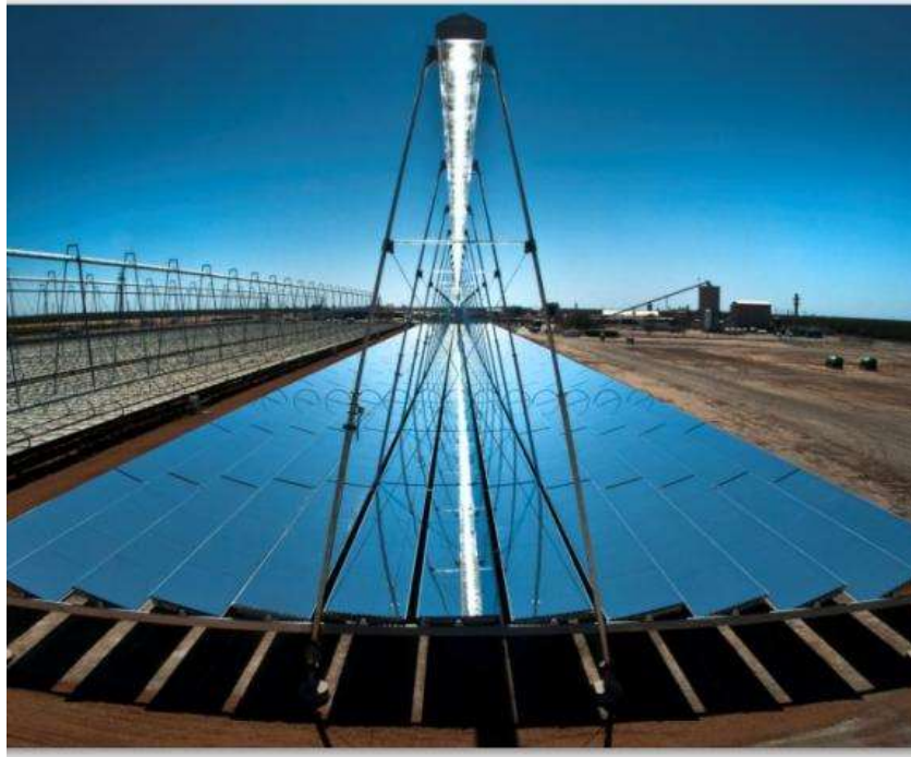
Figure: 2.3.4: Compact Linear Fresnel Reflector
