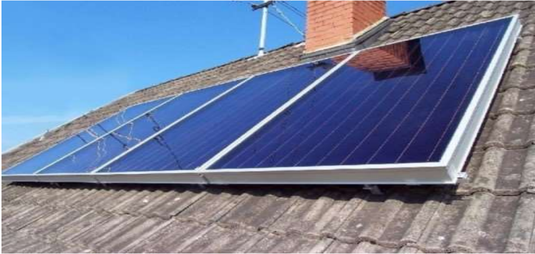
Figure 2.3.1: Flat Plate Solar Collector
