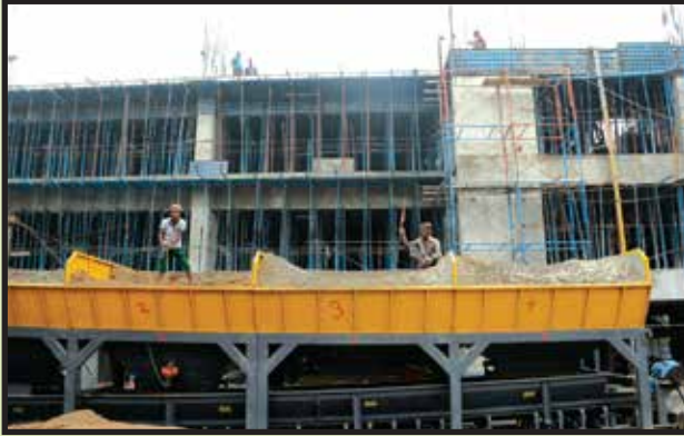
Construction of Utility Building
