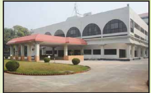
Renovation of Building No-505 has been done
