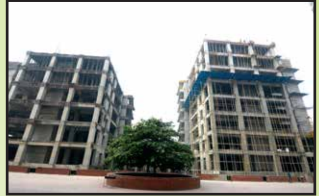
Construction of Tower Building-3 & 4
