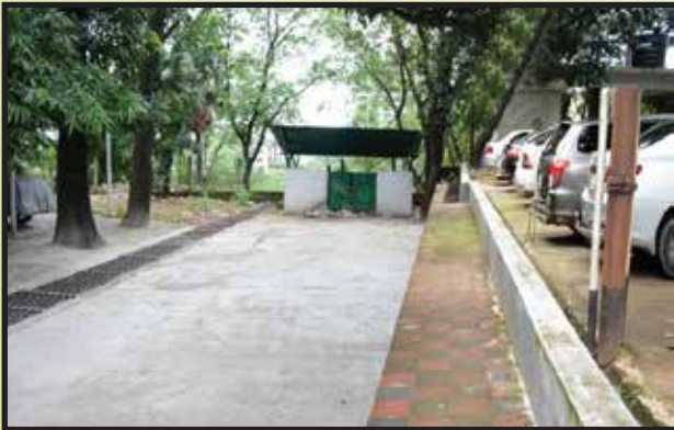
Construction of Hard Standing Road (Near Building No-14) has been done
