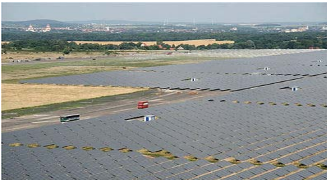
Fig: 2-19. Waldpolenz Solar Park, Germany
