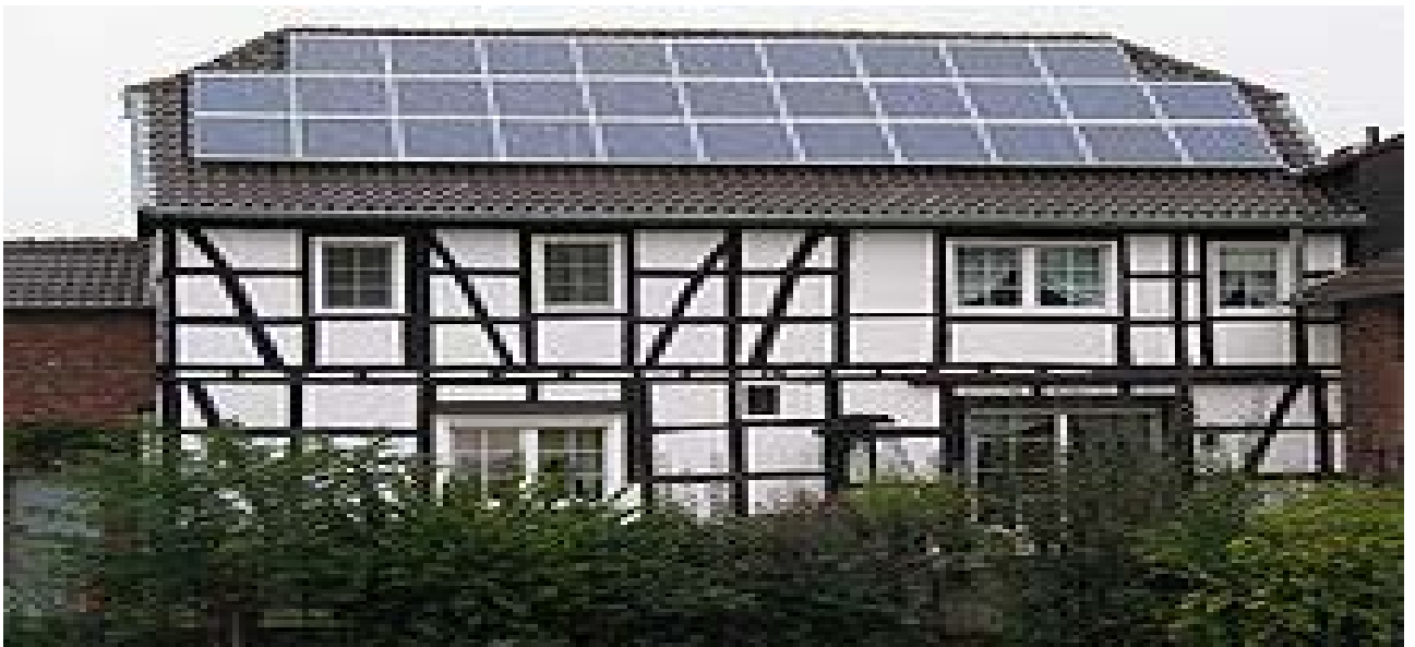
Fig: 2-18. Solar cell array on roof top
