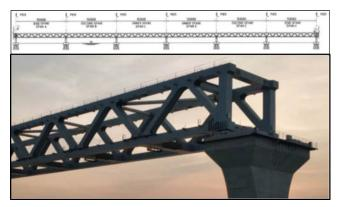
Figure 10: Spans of PMB
