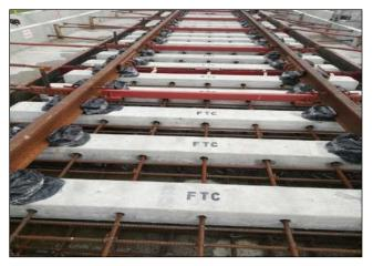
Figure 14: Semi precast cast in situ BLT
