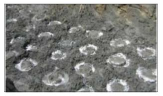
Figure 9: Cement Mixing Piles after construction
