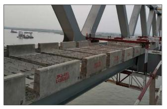
Figure 13: Long Sleeper Embedded BLT over Padma Bridge
