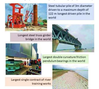
Figure 3: Record-breaking works of Padma Bridge Project (Padma Multipurpose Bridge Project, 2022)
