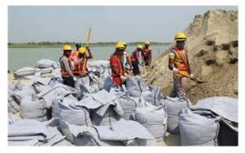
Figure 9: Dumping of Geobags on the lower slope
