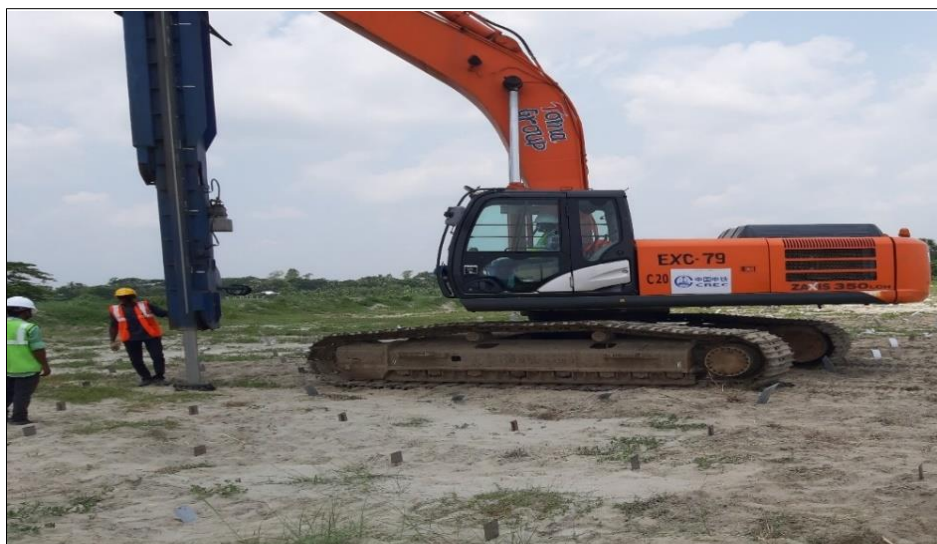
Fig. 3.10: Installation of prefabricated vertical drains in the study area.
