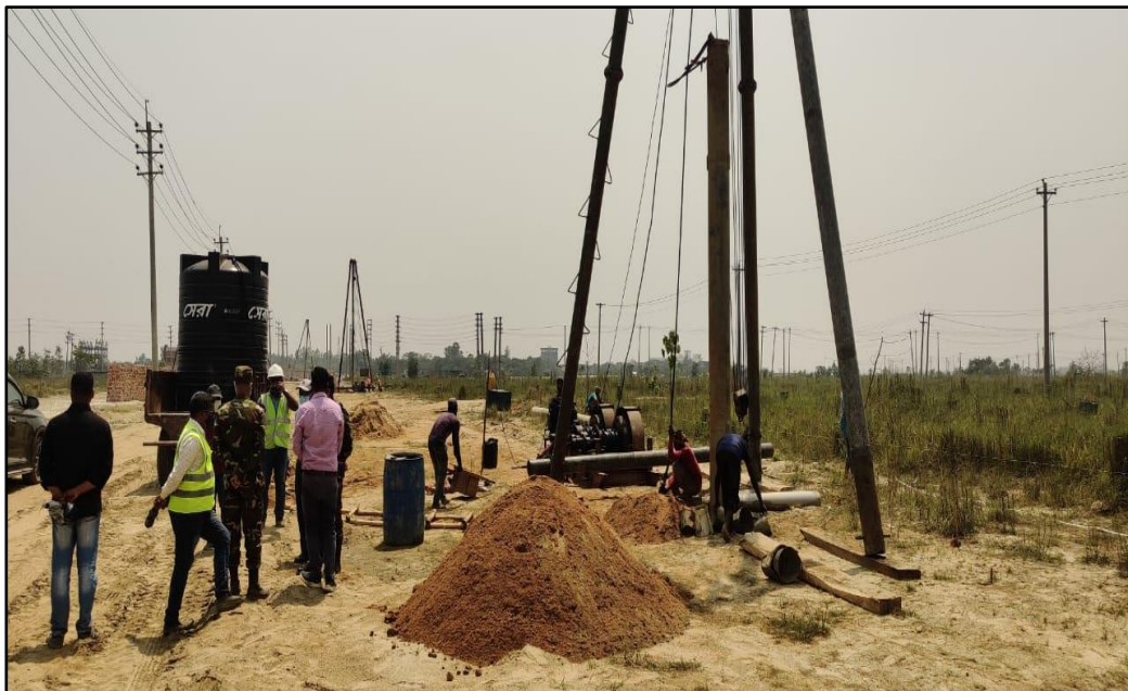
Fig. 3.9: Installation of sand compaction pile in the study area.
