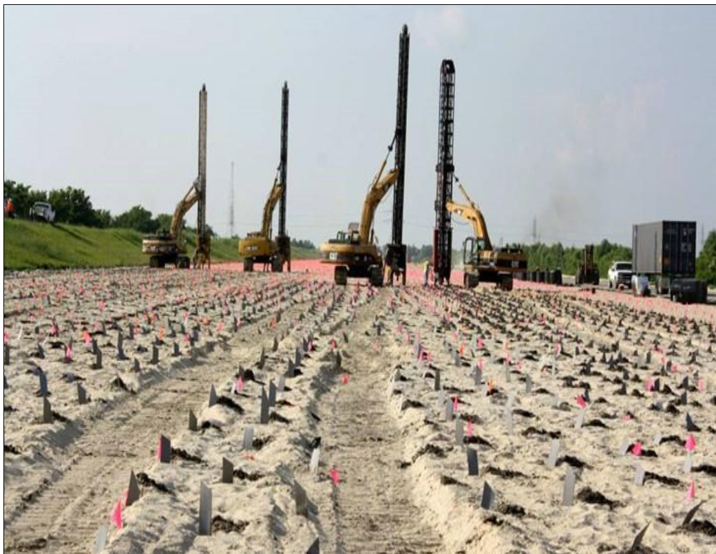
Fig. 2.10: Typical prefabricated vertical drains (PVD) installation arrangements
