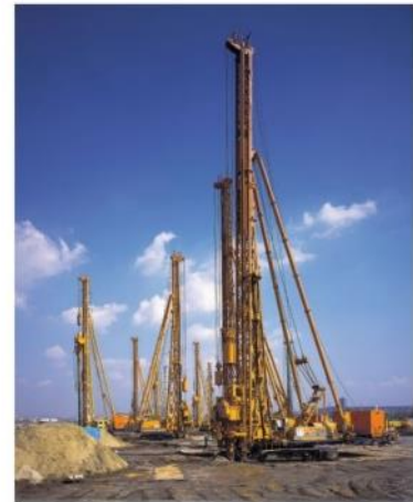
Fig. 2.4: Construction sequence and picture for vibratory SCP (after Ezo, Harada and Otani, 2019).
