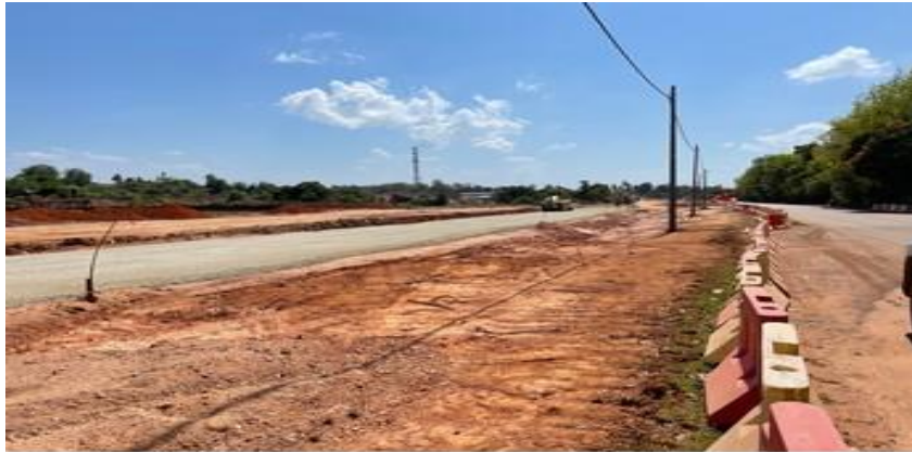
Figure 3.6: Subgrade soil sample from construction site
