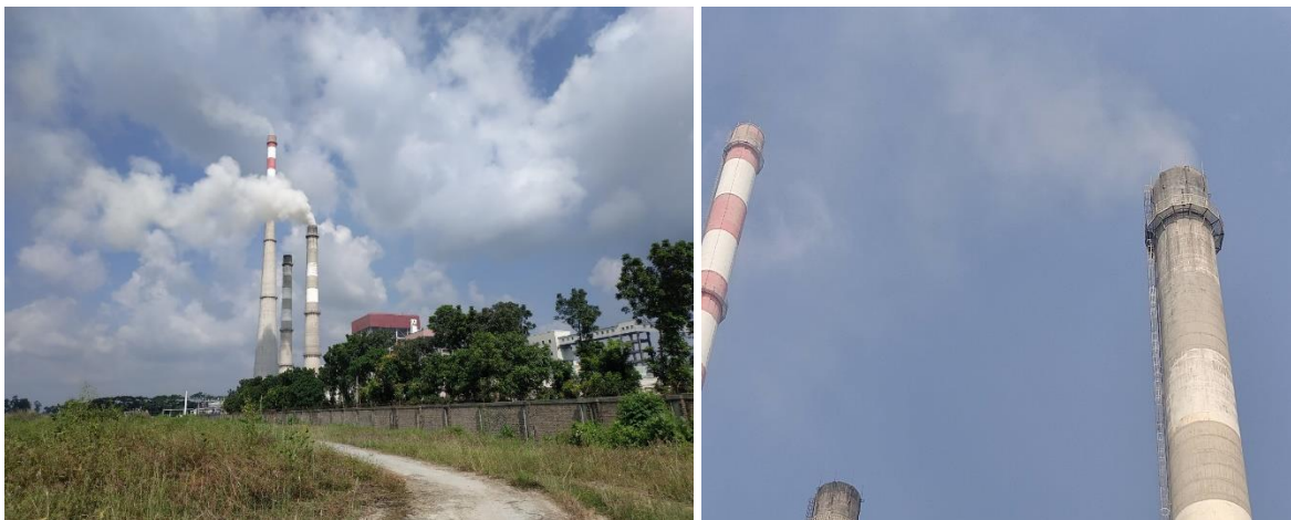
Figure 3.2: Emission from the stack of Barapukuria Thermal Power Plant
