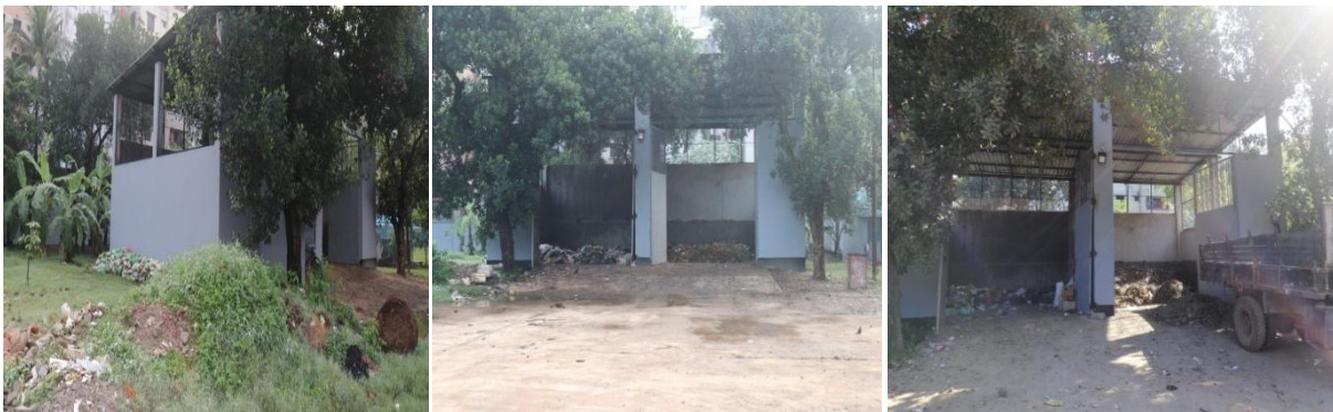
Figure 6.8: Newly established Secondary Transfer Station
