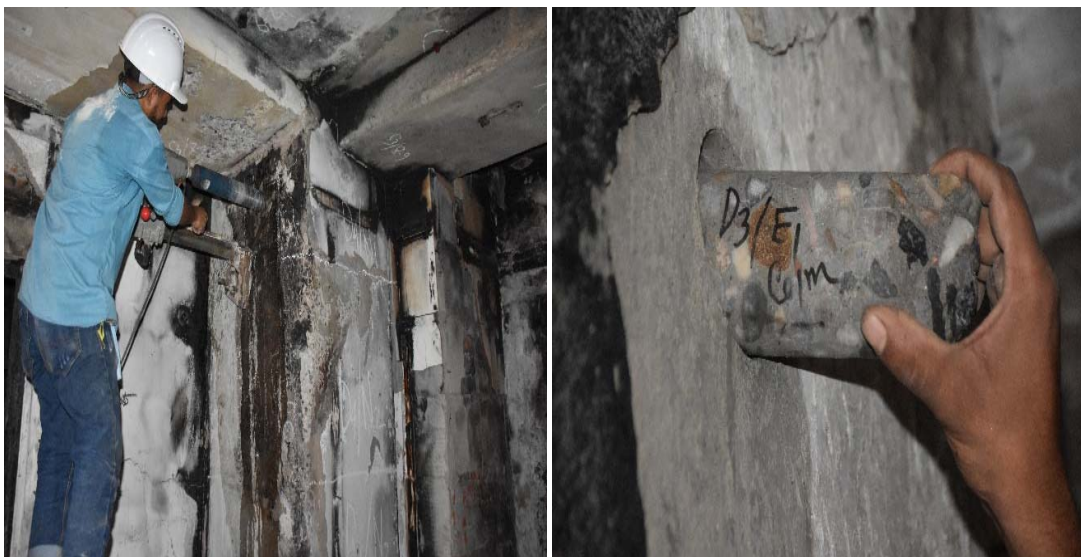
a) Collection of concrete core samples
