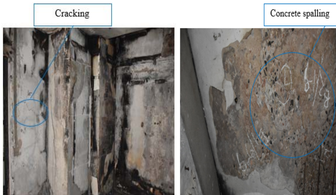
a) The column on the 7 th floor (Grid: D/3)
