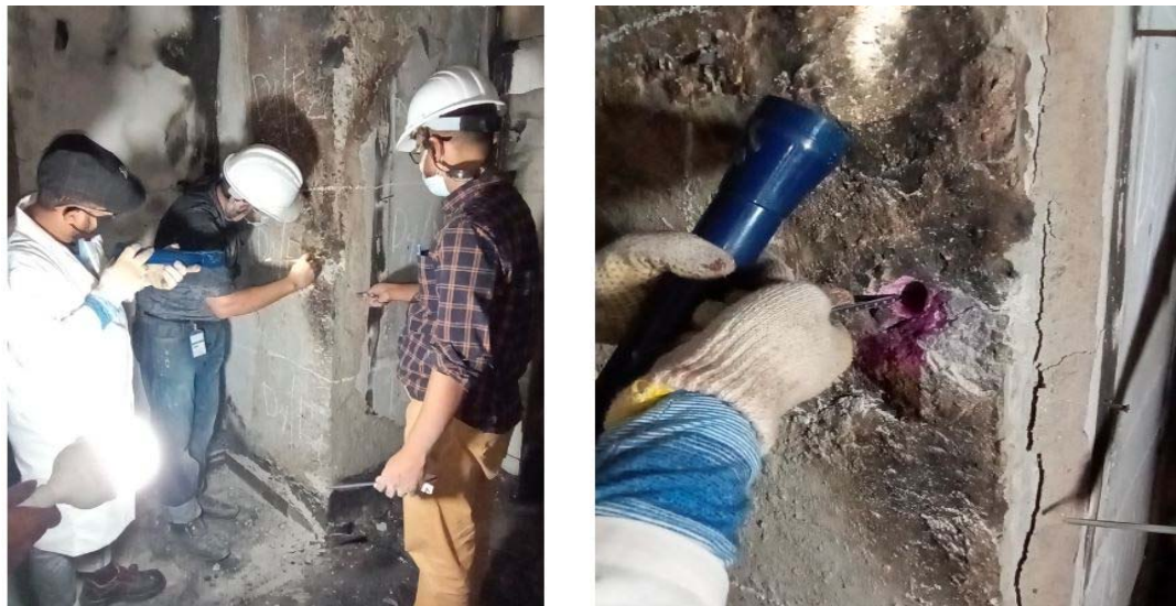
a) Surface preparation for indicator spray b) Measurement of carbonation depth
