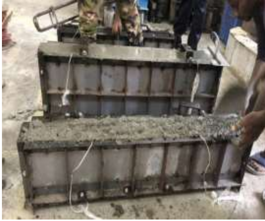
(e) Casting of beams
