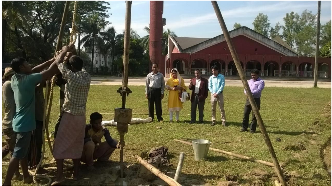
Fig. 3.4: Typical SPT operation.
