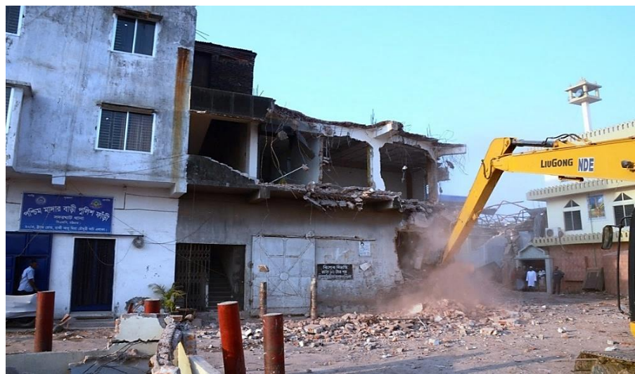
Fig. 1.3: Demolished of an old administrative building in Bangladesh
